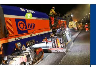
"The high performance of this machine means that we have the capacity to plane the existing surface quicker, which ensures that our Contracting teams can start laying new asphalt sooner to ultimately reduce disruption for road users and drive efficiency for customers."
